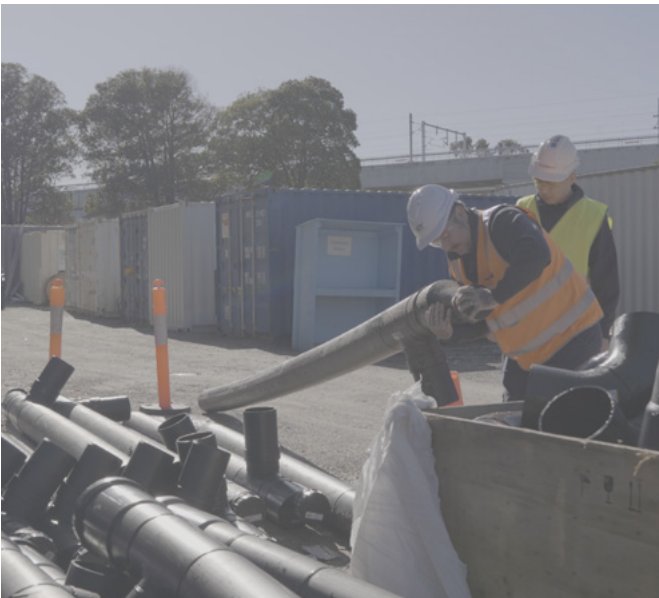
PREFABRICATION ALLOWS OFFSITE ASSEMBLY TO SAVE TIME AND LOWER ON-SITE RISK
