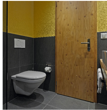
Post-renovation with an upgraded concealed cistern—ready for another 50 years of performance.
