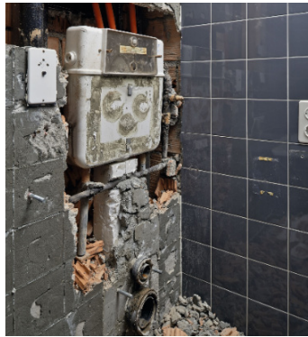
Renovation in 2014 with original Concealed Cistern still in good condition
